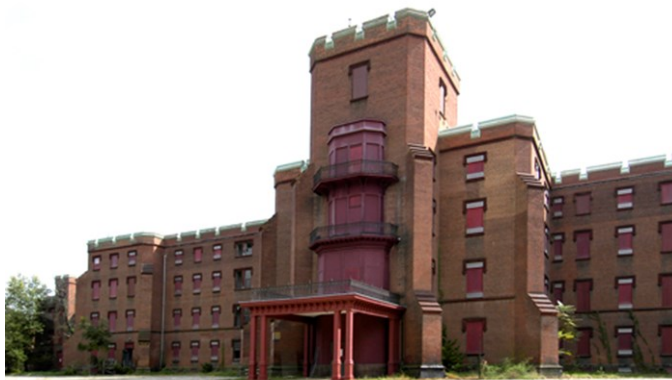
The Center Building is the focus of ONGOING renovations
